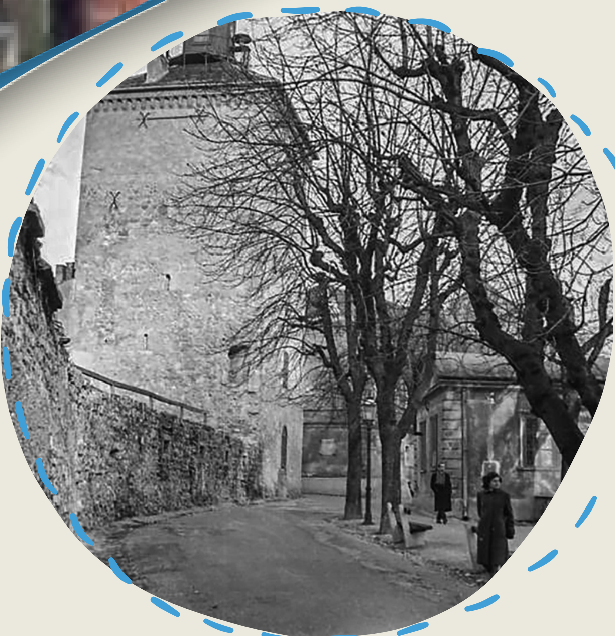
Lotrščak Guard Tower and the Strossmayer Promenade, circa 1960
